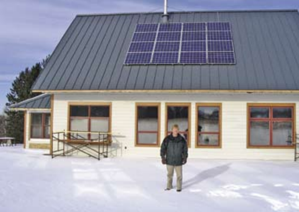
Tom Anderson from Cloquet, Minnesota, stands in front of his 2.53 KW solar-electric system on a sunny winter day.
