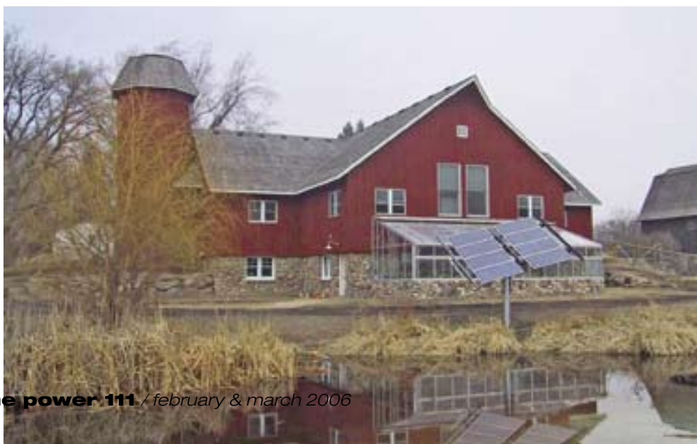
The Dodge Nature Center in West St. Paul, Minnesota, features a 1.0 KW system on a single-axis tracker.
