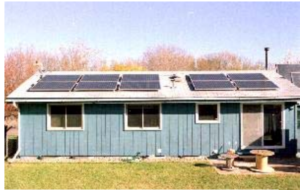
Residential Installation (2.1 kW) Solar Panels in White Bear Lake, MN Photo Courtesy: Solar Electric Power Association
