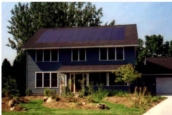
Residential Installation (3.3 kW) Solar Shingles in Northfield, MN Photo Courtesy: National Renewable Energy Laboratory
